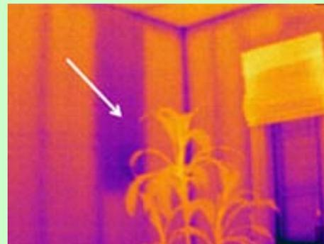
Can you see the missing insulation in this wall?
